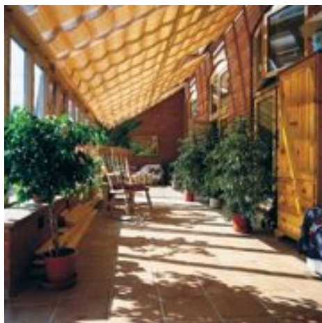
The conservatory that allows maximum passive solar gains © Hockerton Housing Project
